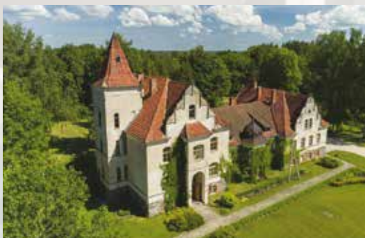
The Mēri Manor house, Bilska Civil Parish.
