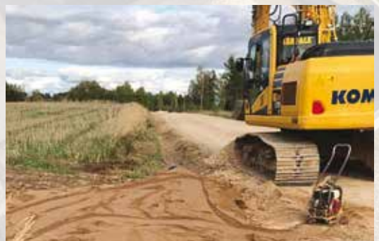
Road construction, Ltd. "8CBR".
